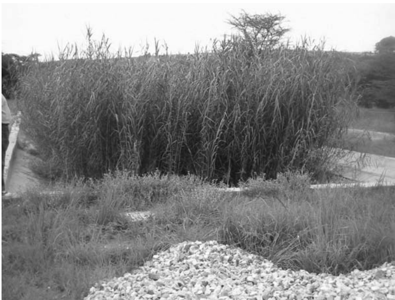
FIGURE 6.3 (See color insert.) Constructed wetland in Tanzania. A high density of plants are selected in the design phase to ensure a high treatment efficiency. The selected plants species are local wetland plants.
