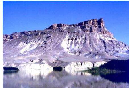
Fig.4 An earth dam in AL-Badia
