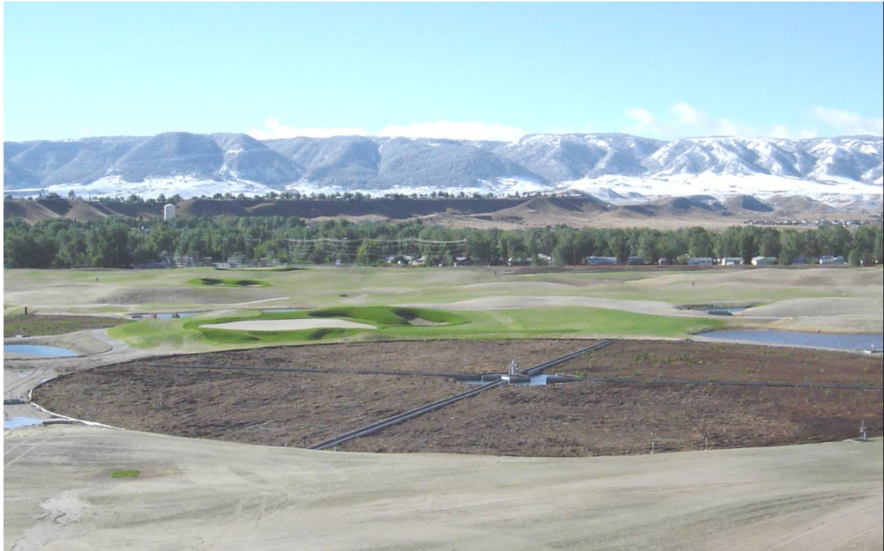
Figure 5. Aerated wetland for groundwater remediation in Casper, Wyoming U.S.A. Photo taken post-construction 2003, North American Wetland Engineering.
