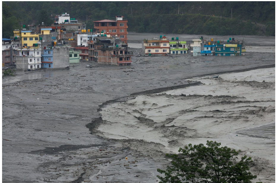
Houses partially buried in sediment as a result of flash floods on the Melamchi River, Nepal, June 2021. Credit: REUTERS / Alamy Stock Photo
