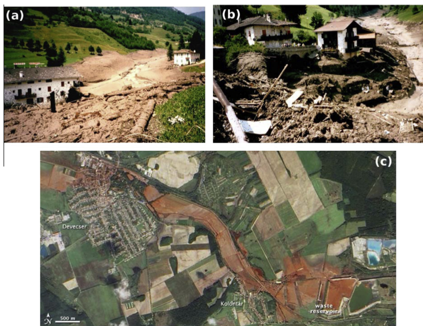
Fig. 4. Photographs of tailings impoundment failures and effects. (a) and (b) Views downstream of the effects of the tailings dam failure at Stava, North Italy, 1985. Used with permission from the Archive Stava 1985 Onlus Foundation – www.stava1985.it . (c) Red mud spill at Akja, Hungary, 2010. Image used courtesy of NASA.
