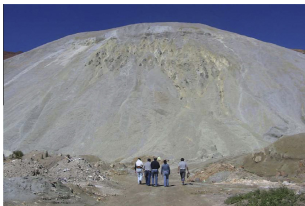
Fig. 5. A portion of the Pailaviri tailings deposit which lies within the Huayna Mayu watershed, Bolivia. The Pailaviri tailings are less than 100 m from Huayna Mayu, which drains to the Ribera de la Vera Cruz, less than 2 km from the location pictured. Such tailings piles are also highly susceptible to wind transport. From Strosnider et al. (2008), used with permission from W.H. Strosnider.
