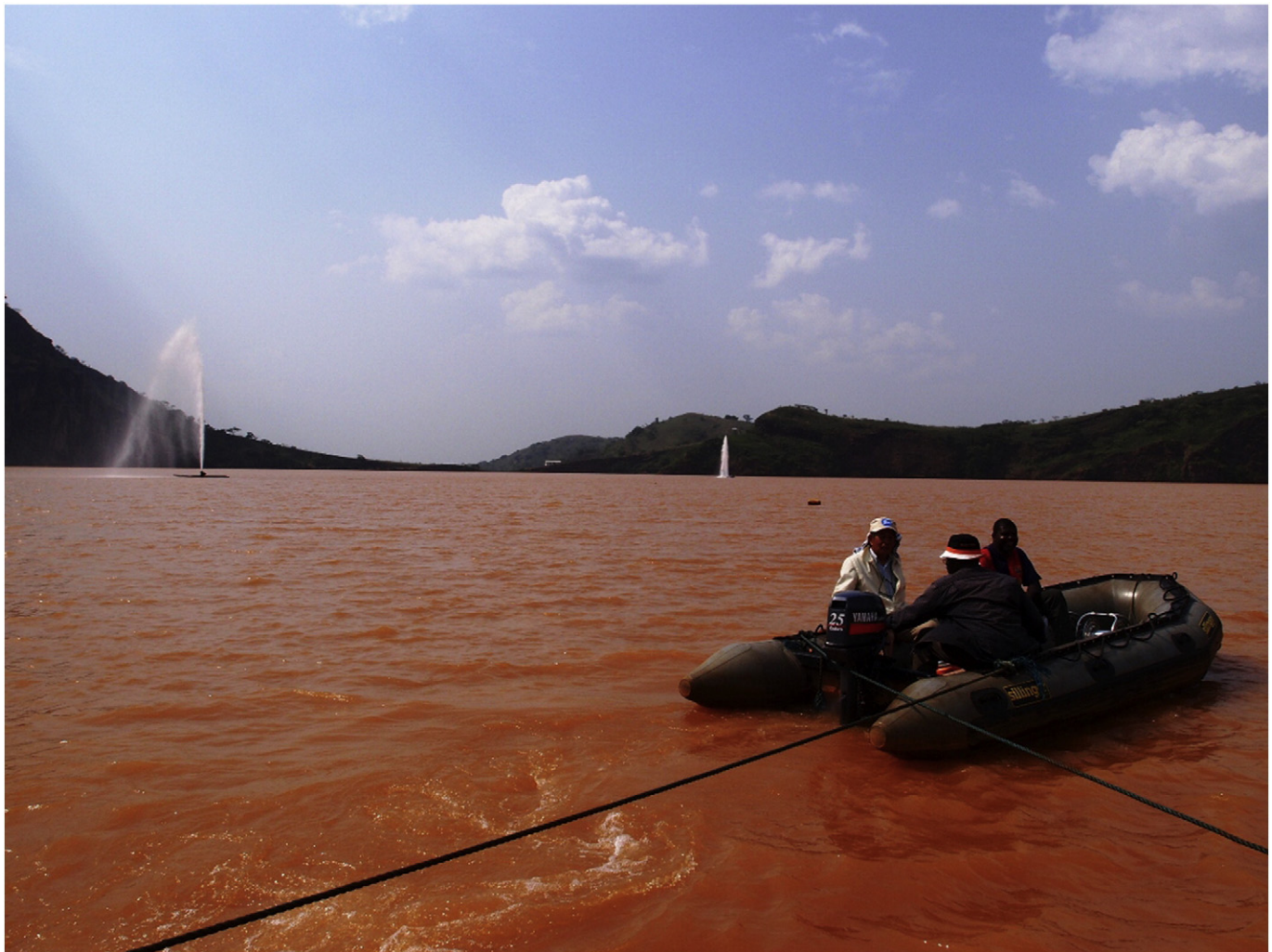
Fig. 7. Degassing pipes in action at Lake Nyos, Cameroon. Deep lake water is fountained to the surface in order to liberate CO 2 . Lake surface water turned red by iron oxide after oxidation of iron dissolved in bottom water, contemporaneously pumped to the surface (picture by Y. Yoshida).
